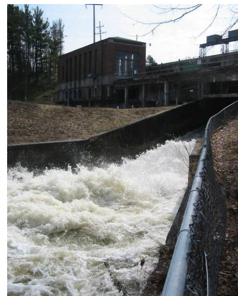
Water roars through the spillway at the Cass Road dam which forms Keystone Pond.
